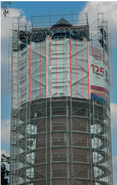
Circular scaffolding at a historical water tower
