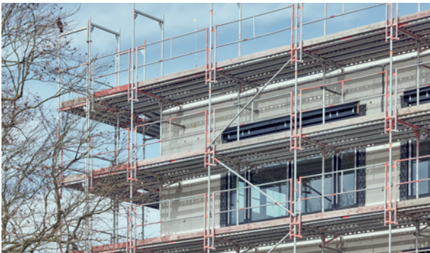
Facade scaffolding, 1.09 m wide, with internal console brackets and I-Guardrails
