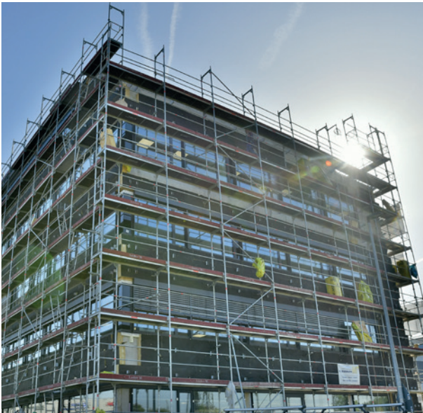
Facade scaffolding at an office building
