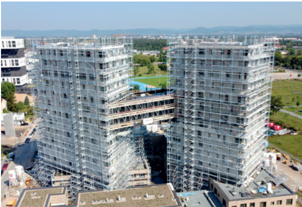
Facade scaffolding at a big apartment area
