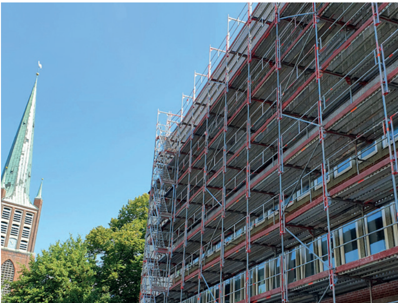
Facade scaffolding at an office building with platform stairway and I-Guardrails
