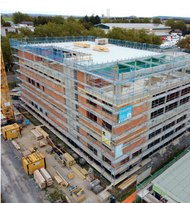
Facade scaffolding with edge protection at an industrial building
