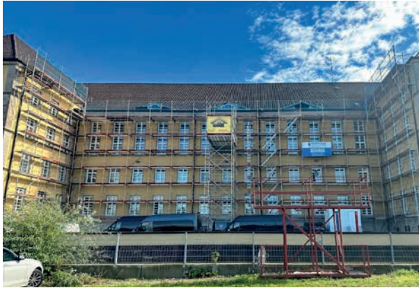
Facade scaffolding with roof edge protection
