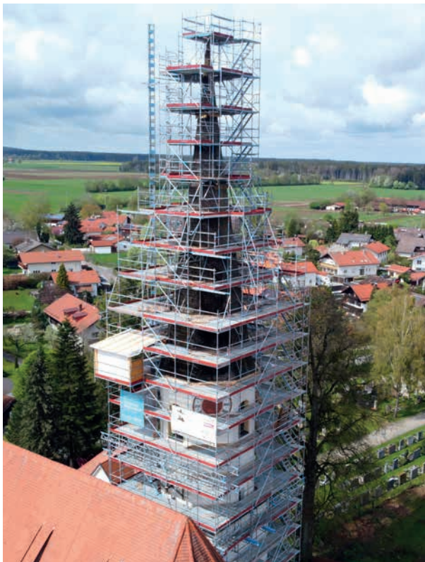
Scaffolding at a church bell tower with flexible geometry adaption and integrated platform stair
