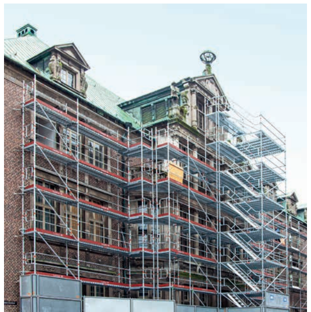
Facade scaffolding with integrated stairtower and access protection enclosing
