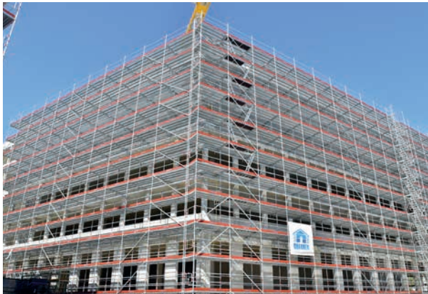
Facade scaffolding with 1.09 m bay width and with external platform stair
